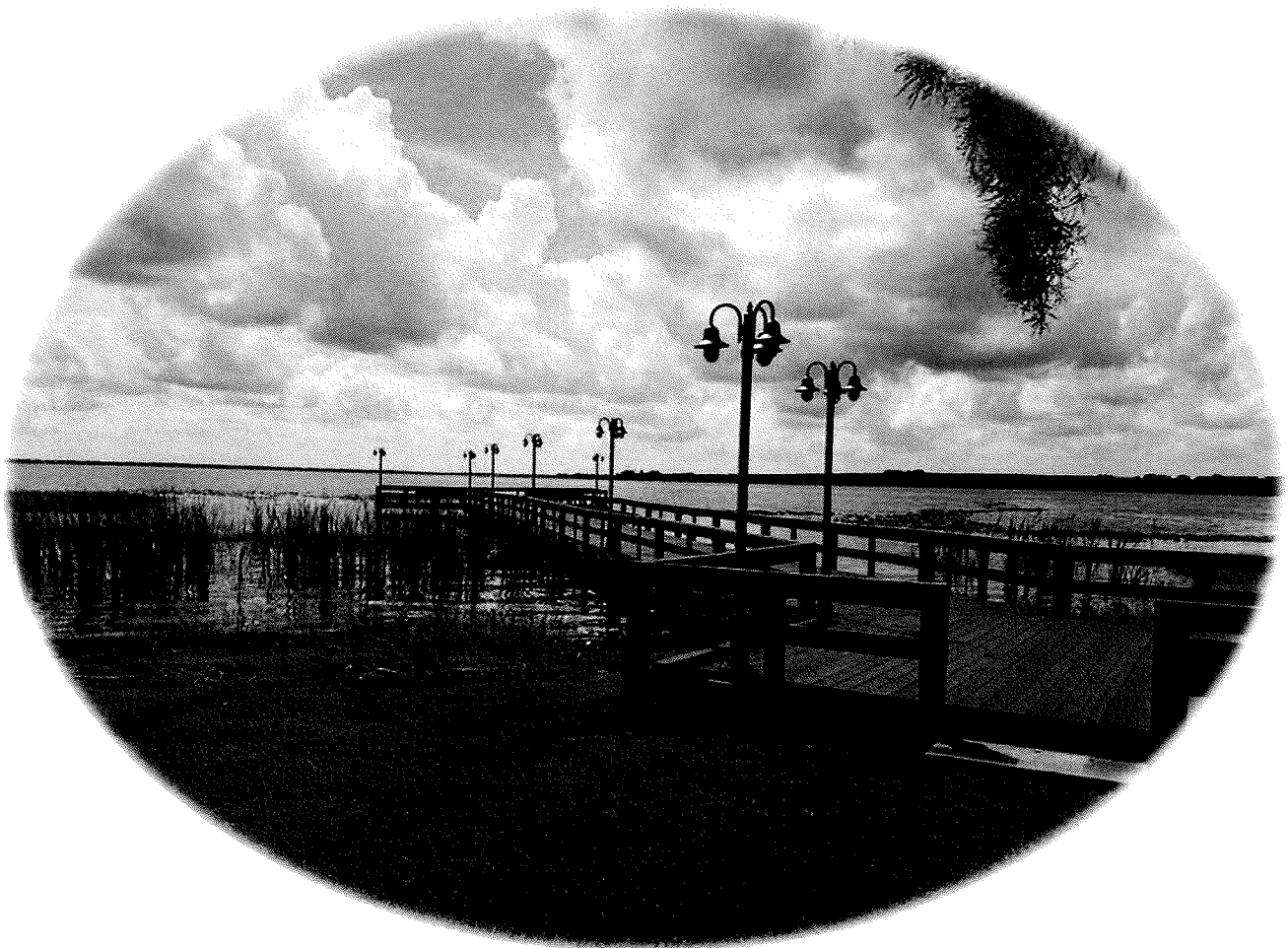
Lake Reedy Pier after renovation
