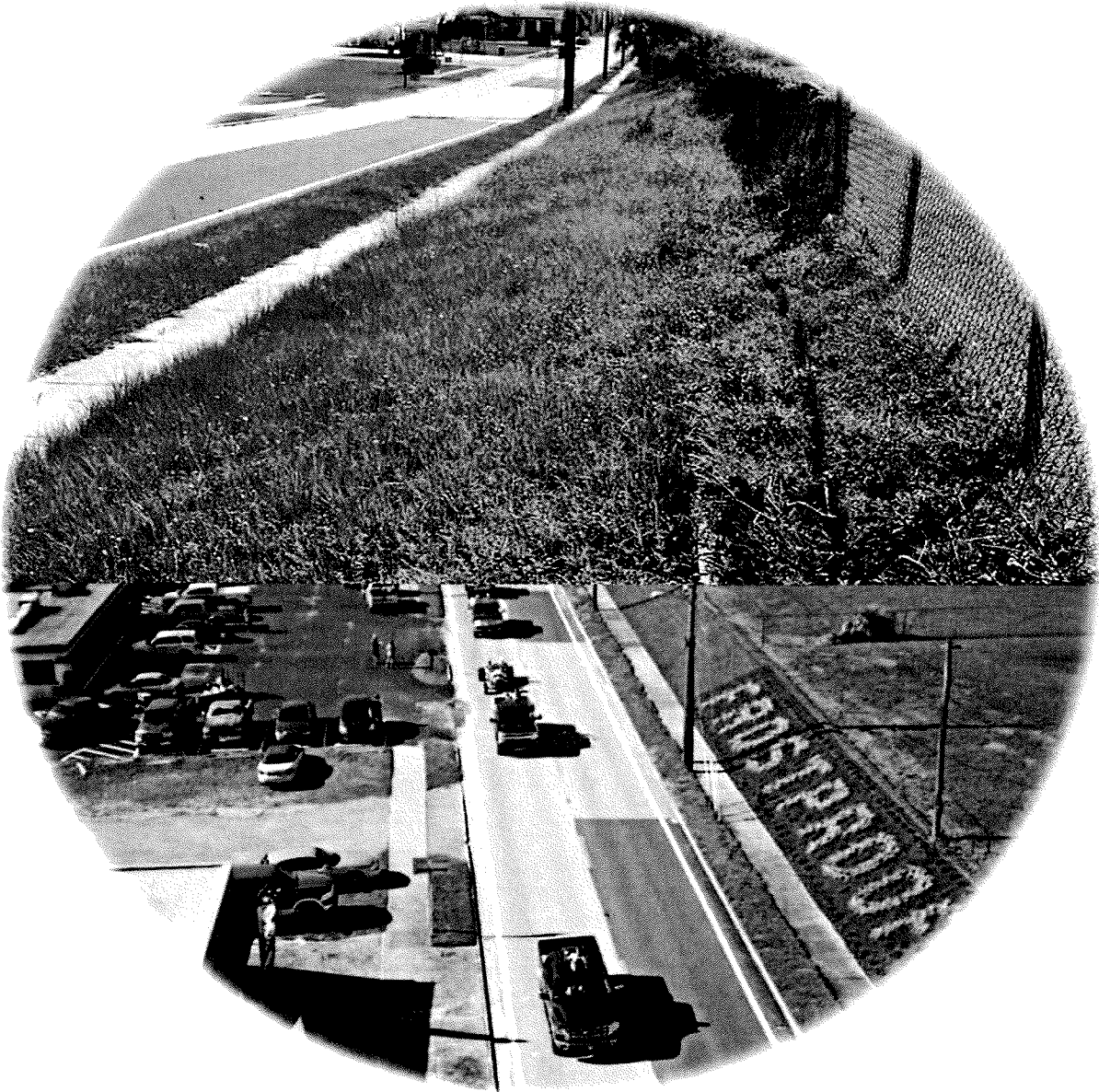
Frostproof Post Office Hill after renovation
