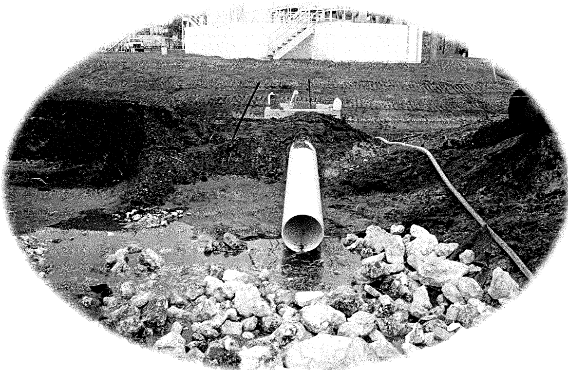
Wastewater Treatment Plant Storm Pond
