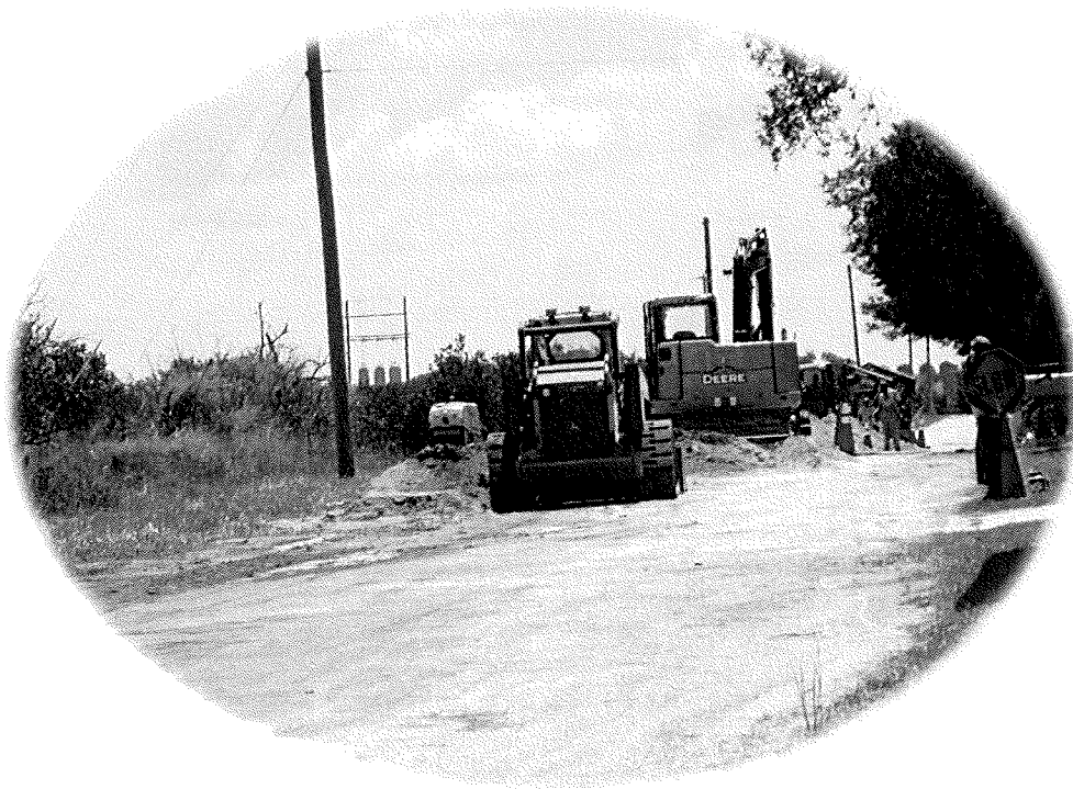
Waterline Loop Project
