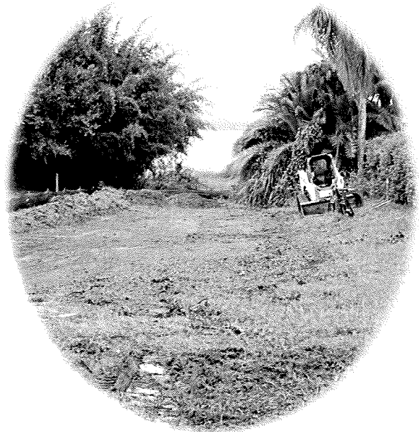
Stormwater Project Wall Street at Lake Clinch
